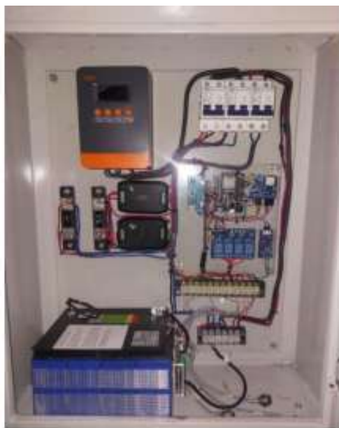
Figure 4. Installation of components inside the control panel
